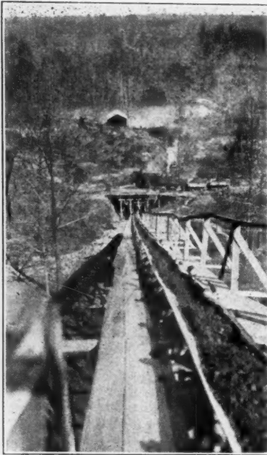
The Conveyor to the Plant
